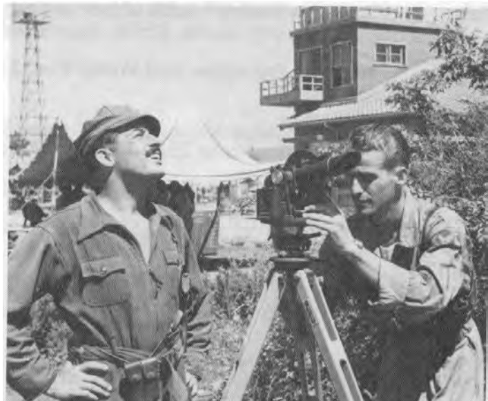
Figure 3-5: AWS’ first Korean War casualty, 1Lt David Grisham, watches Pibal at forward base in Korea in late June 1950 while 20 th WS 1Lt John t. Gordon operates theodolite.
